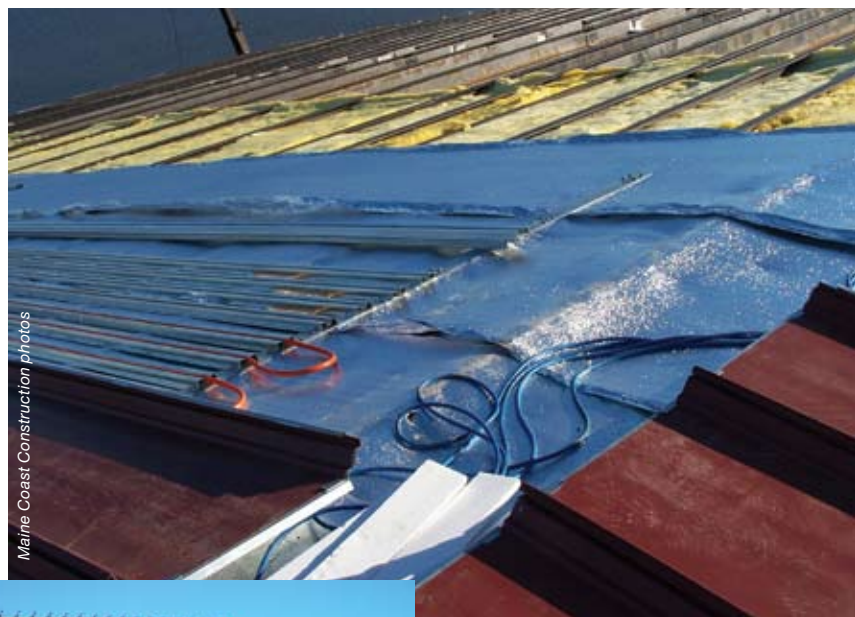
Top: The Dawn Solar system as it appears under the standing seam roofing.
